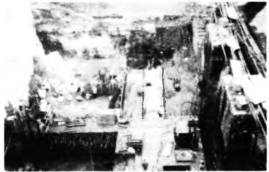
Fig. 1. Photo showing the power house foundation blocks 1-4 under construction
