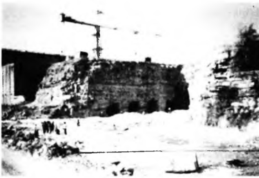
Fig. 5. Photo showing the downstream portal of the tunnels I, II, III & IV
